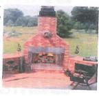
It must have enclosed sides made from bricks, blocks, stone of some type, heavy gauge metal, or some other District-approved non-combustible material, and be built in such a way that the pit becomes a permanent structure. Contact (502) 574-6000 if you are not sure if your planned fire pit meets APCD specifications.
